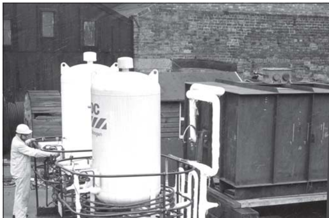
The test tank used to demonstrate viability of polyurethane foam insulation and secondary barrier system at -104°C on Emiliano Zapata
