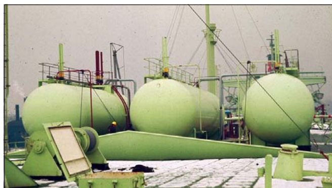
Deck storage tanks at forward end of Faraday
